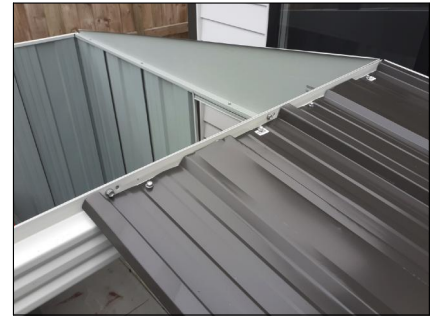
Roof Panels connected to Ridge Beam
