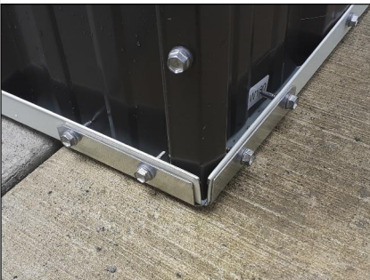
Corner Anchor Exterior - Bottom
